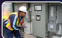
Electrical Safety and Energy Assessment
