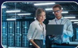
Data Center Assessment
