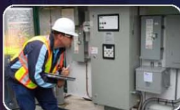
Electrical Safety and Energy Assessment
